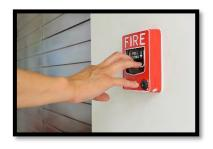
General Description: Fire alarm systems consist of manual and programmable pull stations, visual/audible alarm devices, addressable smoke detector/sound bases and smoke/heat detectors in individual sleeping rooms, corridors, common area and mechanical spaces.
